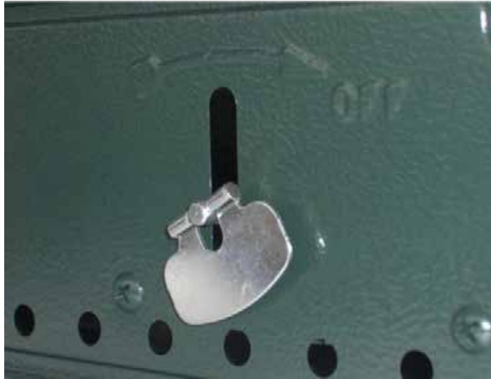
Figure 8 Auxiliary Burner Control
